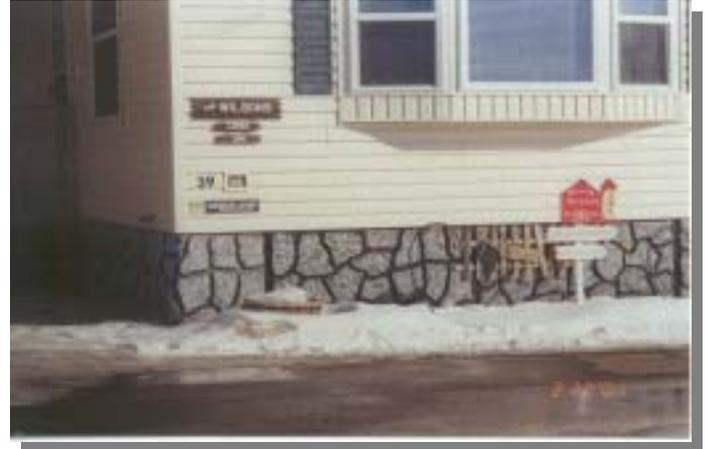
**FIRE:** *StoneSkirt* is made out of concrete and is non flammable. Fake Rock will melt or burn when exposed to a flame.
